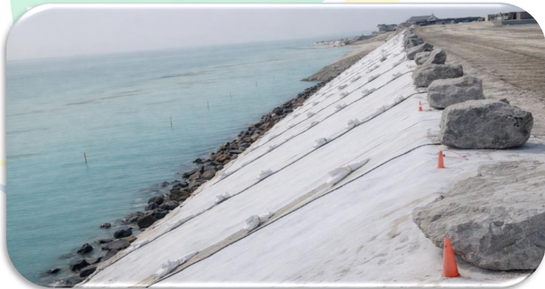
Geotextile Installation
