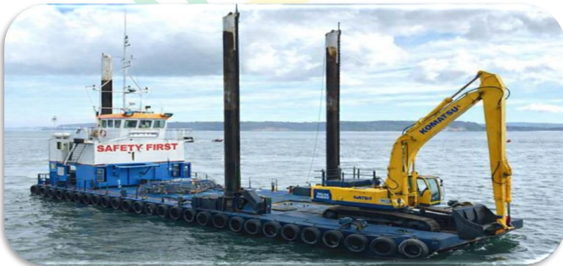
Offshore Barge Works
